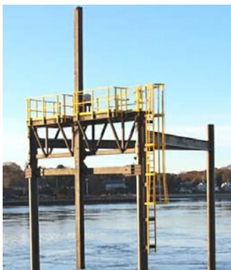
**A tidal current platform in the Cape Cod Canal will soon test its first underwater turbine. (Marine Renewable Energy Collaborative)**
